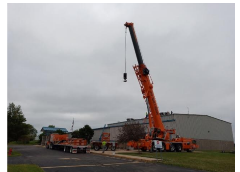
Large crane for HVAC replacement that was completed in July.
